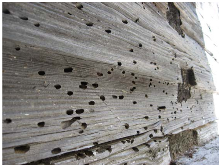
Figure 10: Hylotrupes bajulus flight holes and galleries.
